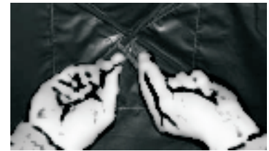
Secure Fiber Poles at Peak of Roof
